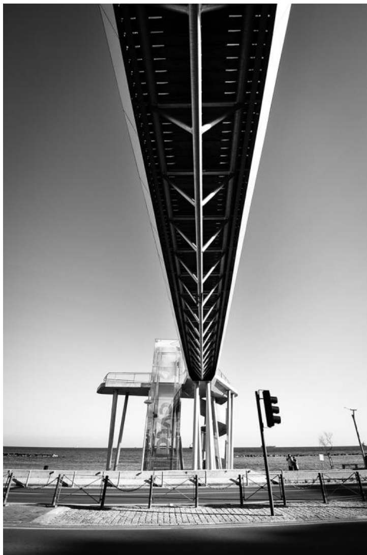
Figure 15. Margarita Danou's CYTA Footbridge in Limassol, 2013 (EU Mies Award 2015)
