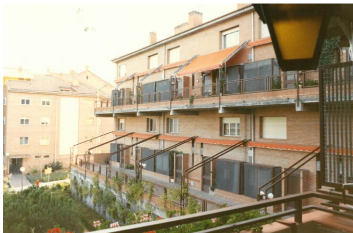
Figure 4. Exterior of the 109 social housing units in Tres Cantos, Madrid, designed and built by Margarita Mendizábal (1978)
