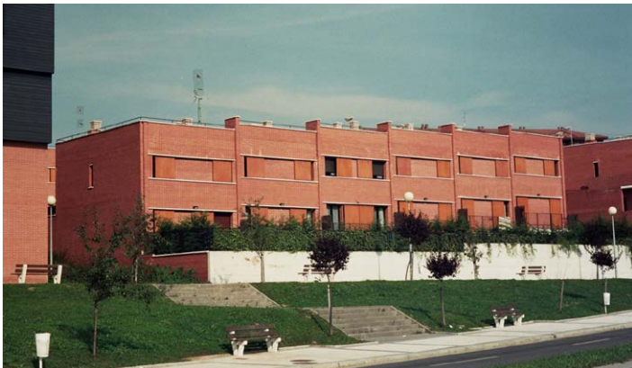
Figure 7. 42 social housing units, Donostia/San Sebastián, Gipuzkoa (1993), Gloria Aríztegui, Antxon Martínez de Salazar, and Lucas Etxebeste
